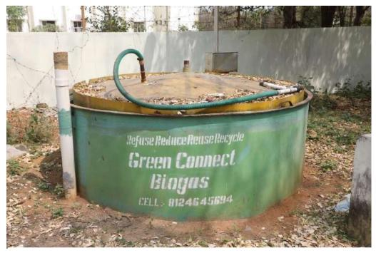
Biogas Plant installed at University Campus utilizing the food wastes of hostels for generating biogas
