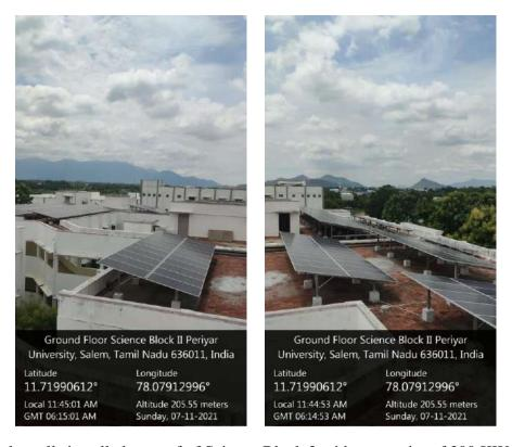
Solar cells installed on roof of Science Block 2 with a capacity of 300 KWs
