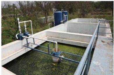
Sewage Treatment Plant with a capacity of treating 120 KLD at Periyar University. Recycled water of about 80000 litres is used for irrigating the landscape.
